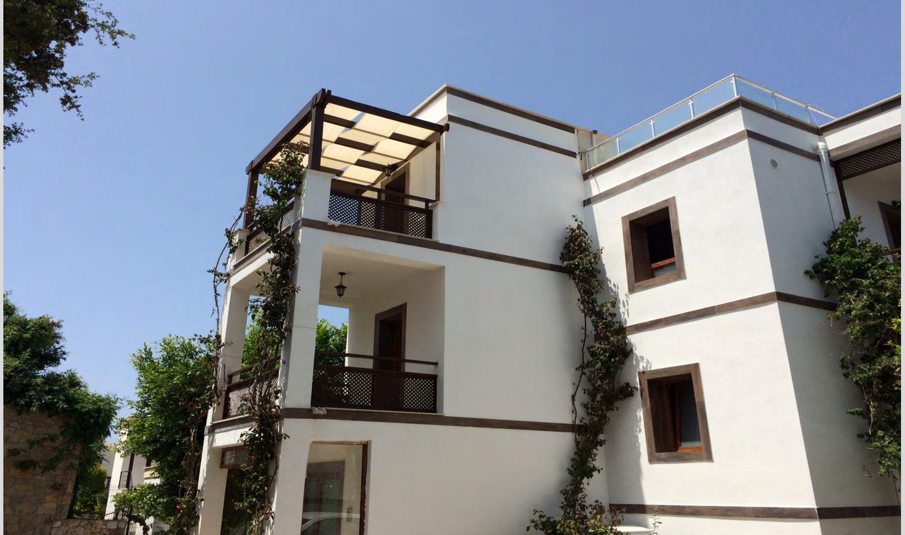
TERA CONSTRUCTION - YALIKAVAK
